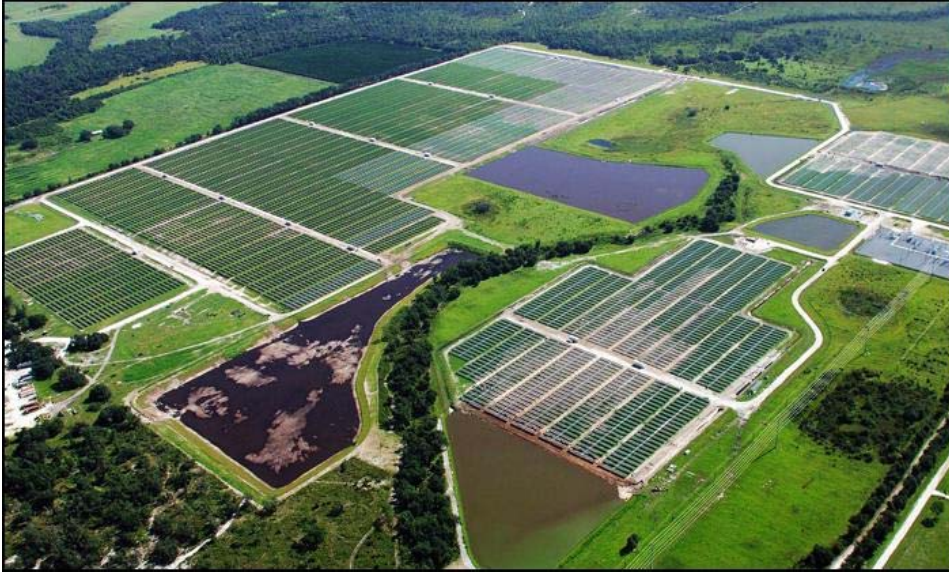
An aerial view of the Desoto Next Generation Solar Energy Center, the largest photovoltaic power plant in the nation. Newkirk Electric Associates, Muskegon, was heavily involved in its construction. It's being visited today by President Barack Obama.
